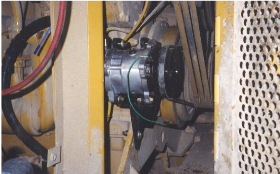
Compressor and mount in place.
