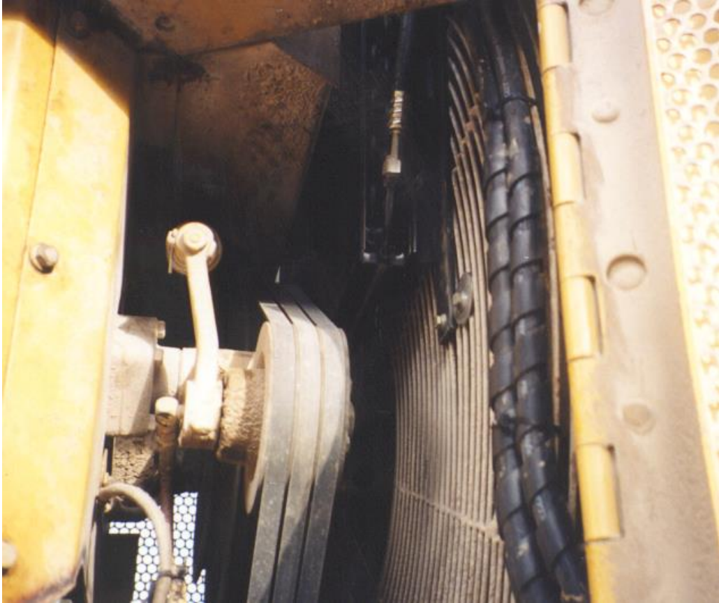
Hose routing up fan screen to condenser.
